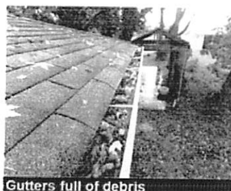
Gutters full of debris
