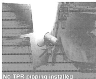
No TPR piping installed
