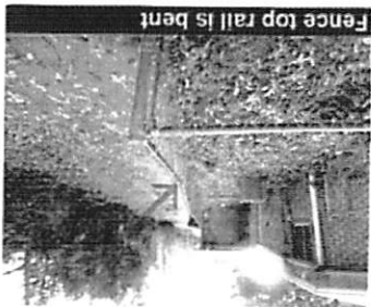
Fence top rail is bent
