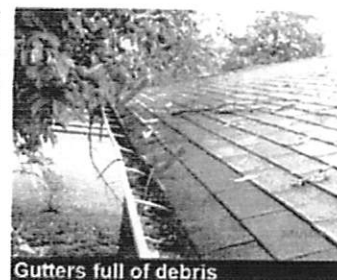
Gutters full of debris
