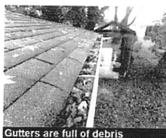
Gutters are full of debris
