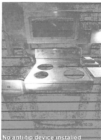
No anti-tip device installed
