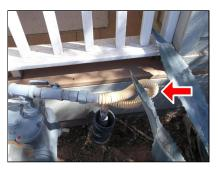
(3) The gas meter is in a traffic corridor and does not have protection to shield it from damage - Review.
