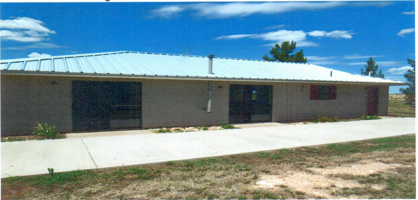
# 3. Rear of home facing East.
