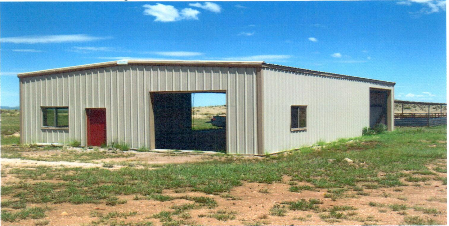
# 5. Metal structure facing South, North of home.
