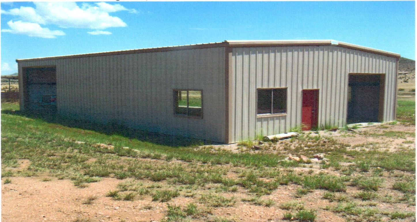
# 6. Metal structure facing West, North of home.
