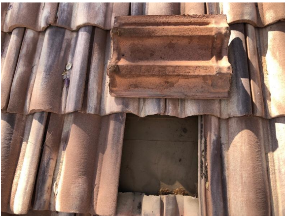
Broken mortar pack
